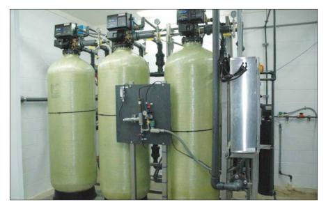
These three vessels used to remove nitrate. Each vessel measures six feet by two feet diameter and contains nitrate selective resin that allows an exchange of chloride for nitrate.
