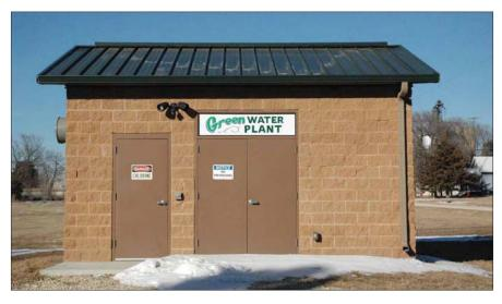
The water system improvement project at Green included this water plant building that houses the nitrate removal units and chlorination equipment.
