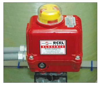
An electric modulation butterfly valve controls the flow from the wells, allowing for the desired blend of raw well water with treated water.
