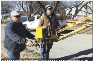
Onaga Superintendent Lynn Krohn and Operator Rick Glessner use the valve exerciser to operate the valve. With the type of valve used in this system, each 6-inch valve required 23 turns to fully close.
