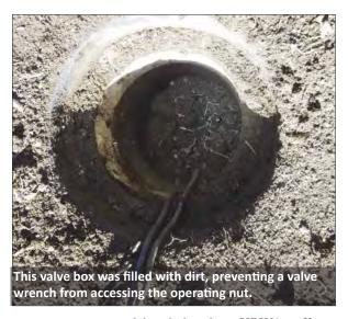
exercising their valves. KRWA staff have been extremely successful in restoring many valves thought to be irreparable back to full function. KRWA's valve exerciser trailer also has a vacuum and power washer to clean out the valve riser boxes or meter pits that have filled with dirt.
