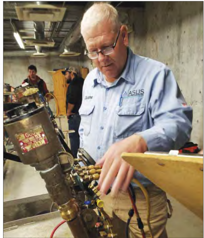
Duane McGowan with Fort Riley Utility Services refreshes skills testing backflow preventers at another training event at Grandview Plaza in February 2022.
