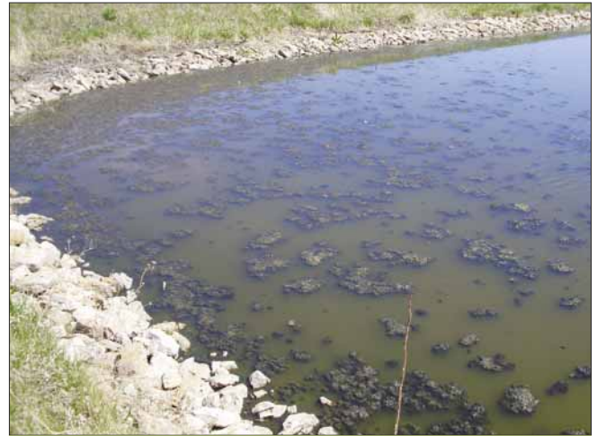
Generally, once a turnover has started, wind will blow the clumps of floating sludge to the corners of the lagoon. Wave action will eventually break up these solids and they will settle back to the bottom of the lagoon.
